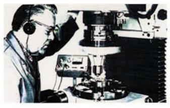
The contact indicator serves for the acoustic and visual monitoring of the grinding process when mach in ingsmall bores (accessory)
